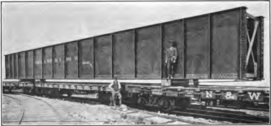
FIG. 114.—Two large plate girders X-braced for shipment on flat cars. (Courtesy of Virginia Bridge & Iron Co., Roanoke, Va.)
